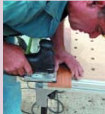
**Use a jigsaw to cut away the bottom 20mm of the tenons on each end of the rails as the mortices are 80mm.**
