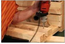
**9.** Fix the back rest strats to the frame with Decking screws (5 x 75mm).
