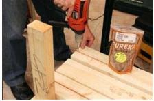
7. Turn the bench over and start fixing the seat slats to the frame with Decking screws (4.5 x 60mm)
