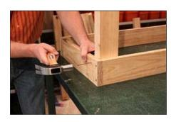
**2.** Attach the front feet to the frame on either sides with Decking screws (4.5 x 60mm). TIP: use a hammer to knock in the decking screws a bit before driving them in wit a power tool. This keeps the decking screw in place.
