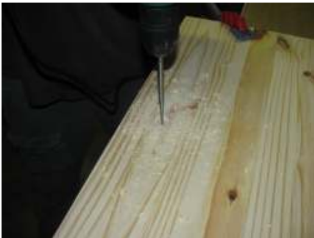
Item 3.7 Drilling of hole in lid for finger hole
