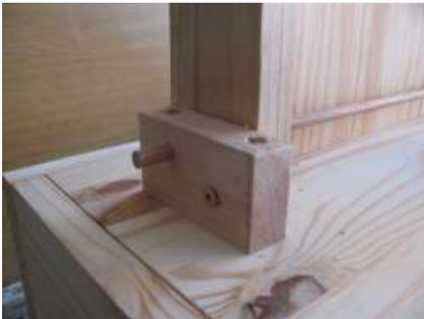
Item 4.15: Dowel keeping flap in position
