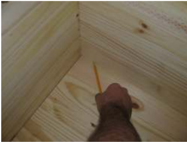
2.8 Marking for positioning of strips
