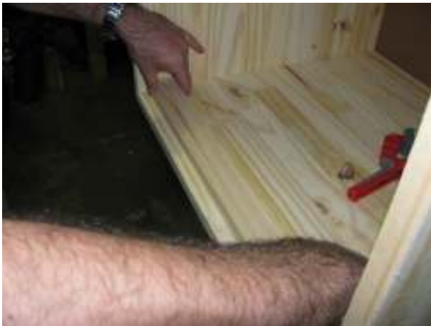
Item 3.2 Placing of sides for lid to fit onto on the long length
