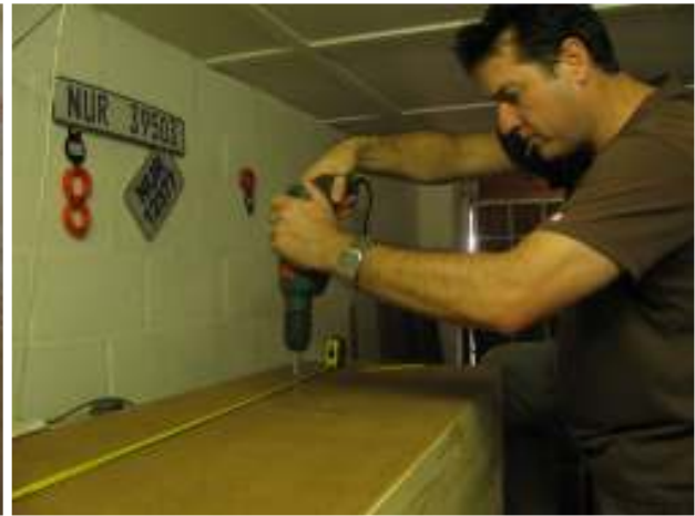
2.9 Fixing of bottom sheet
