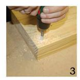
3. Use a 10mm Eureka Wood bit to drill holes at the four marks in all three of the planks.
