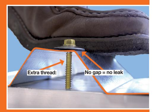
The top section of thread pulls the roof sheeting tightly against the bonded washer, ensuring a watertight seal and better load bearing capability.
